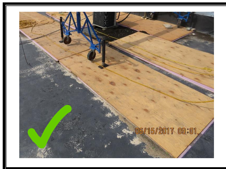
Inadequate roof protection – the plywood corners could damage the roofing
