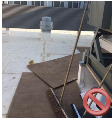
Inadequate roof protection – the plywood corners could damage the roofing
